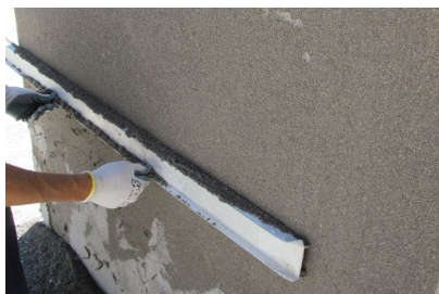
Levelling of surface with ruler
